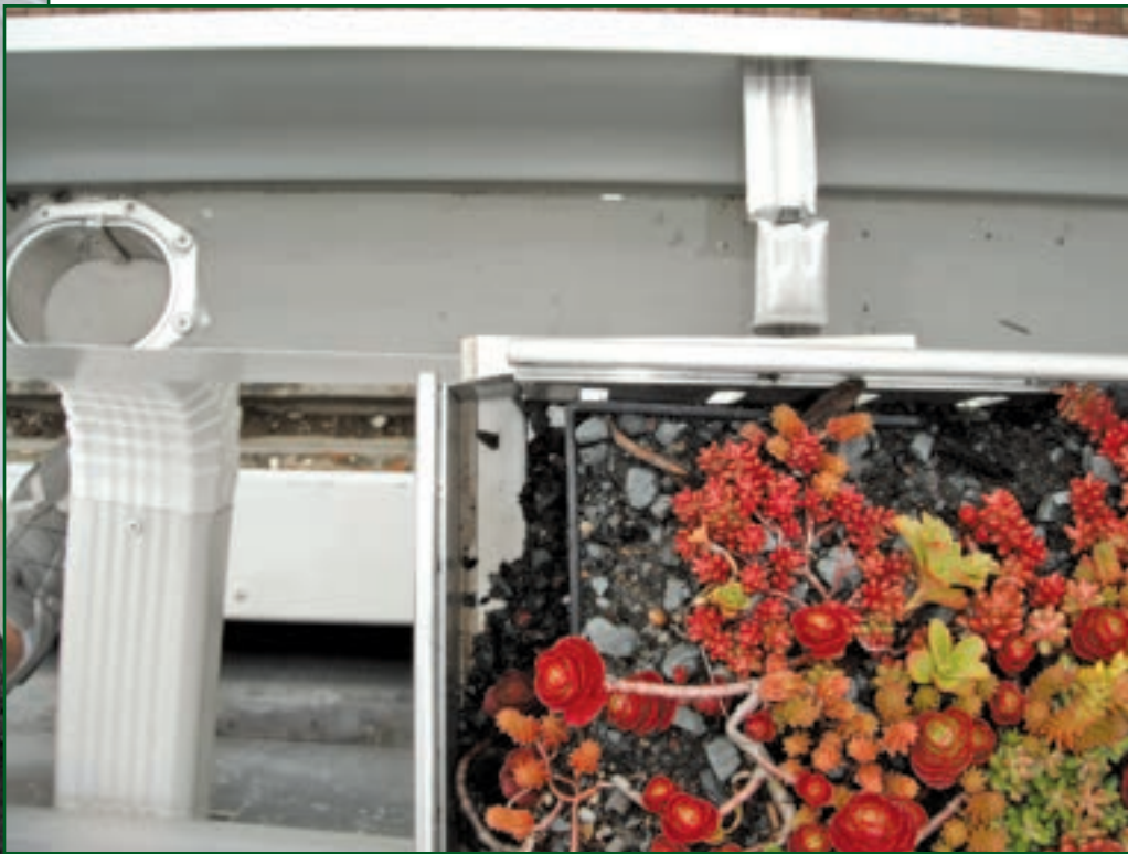
Figure 2. Draining edge detail.
