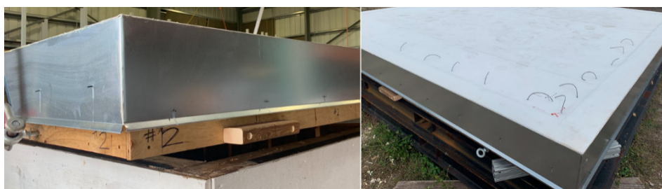
FIGURE 8. Photos showing pressure taps. The left photo shows outermost pressure taps on the fascia. The right photo shows the pressure taps for the membrane. Note: the pressure taps were trimmed flush to the fascia and membrane prior to testing.
