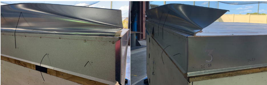
FIGURE 13. Photo of failure mode of Configuration #3 up close.
