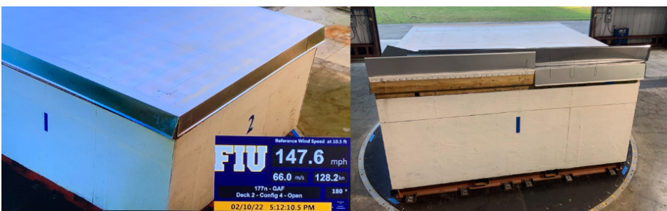
FIGURE 14: Photo of failure mode of Configuration #4.
