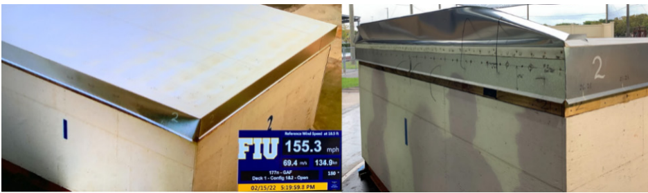
FIGURE 11: Photos of failure mode of Configuration #2.
