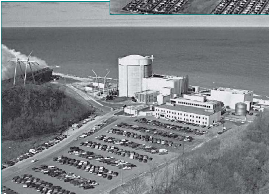
Figure 3 – Example of Exposure D: a building at the shoreline (excluding shorelines in hurricane-prone regions) with wind flowing over open water for a distance of at least one mile. (Photo courtesy of American Society of Civil Engineers.)
