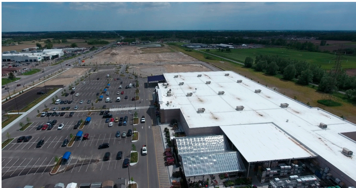
Figure 2. An example of a big box retail store, with a reflective roof membrane.
