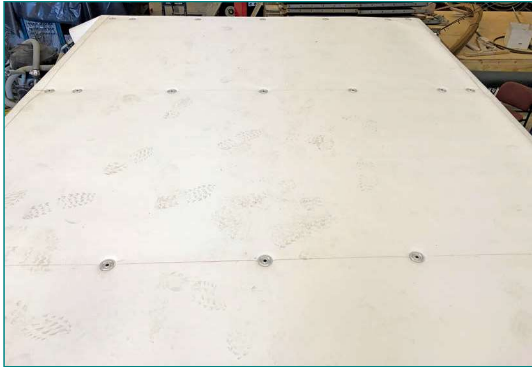
Figure 3 – The installed TPO for Test #2.
