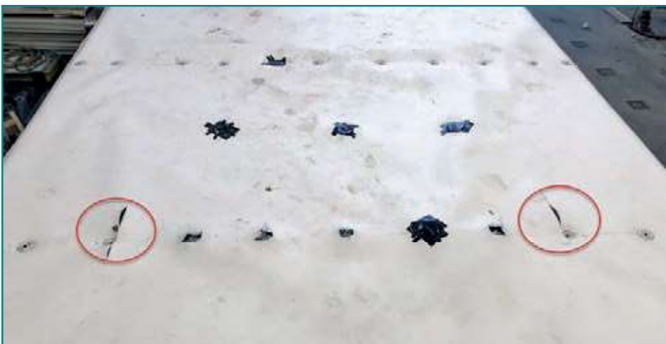
Figure 6 – The outcome of Test #1. The membrane ruptured at the center row of fasteners. The outer two fastener locations where the membrane tore in an “L” shape are identified by red circles.
